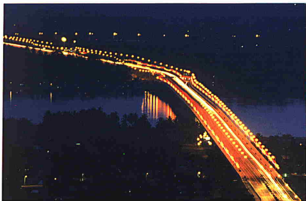
The Sultan Mahmud Bridge which spans across the Terengganu River is the second longest in the country.
