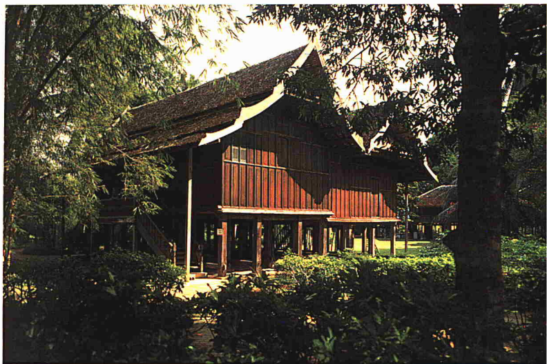
The old palaces in Terengganu, such as this, resembles large houses of Malay architecture from the outside. However closer inspection will reveal its ornately carved woodwork. Although many of the palaces were built more than a century ago, only minimal work was needed to restore them to their former glory.
